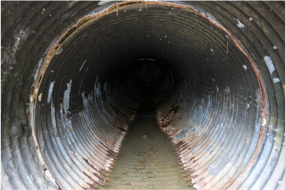
Photograph 3 – Pipe at Outfall 003
